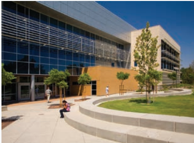
CSU Bakersfield Classroom and Office III, Bakersfield
