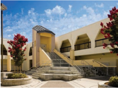
Logan High School New Science Building, Union City
