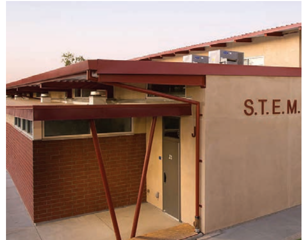
Bella Vista High School STEM Building, Fair Oaks
